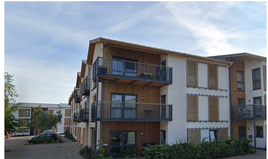
Example of a flatted development with a dual frontage and separate ground floor entrances taken from google streetview
